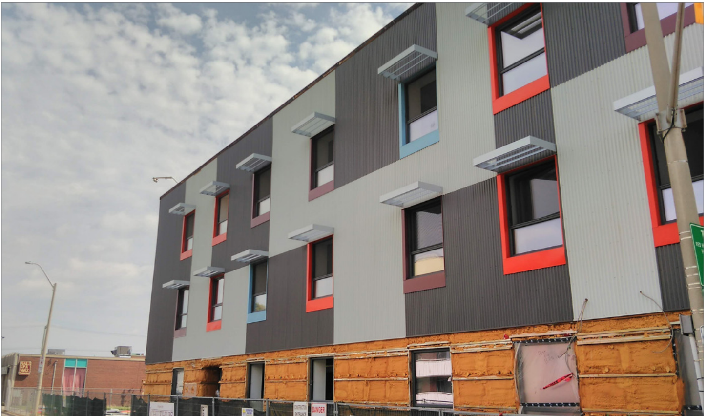
Figure 4 External photo showing triple-glazed windows.
