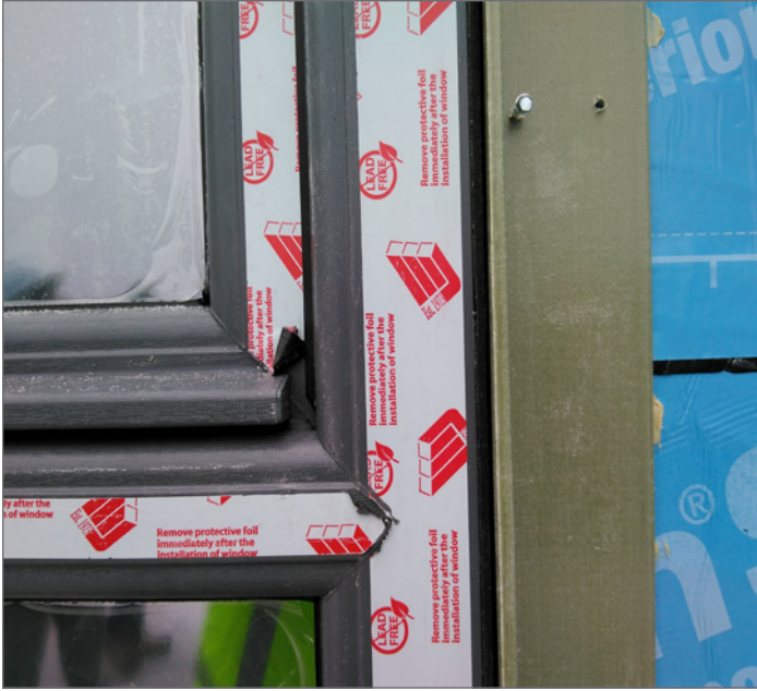
Figure 2 Window detailing for airtightness.
