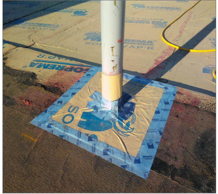
Figure 3 Roofing airtightness well-sealed pipe.
