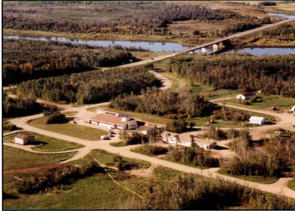
Photo of Muskoday First Nation community facilities. Bottom left: water treatment plant. Center left: administration building. Center right: health clinic. Background: South Saskatchewan River.
