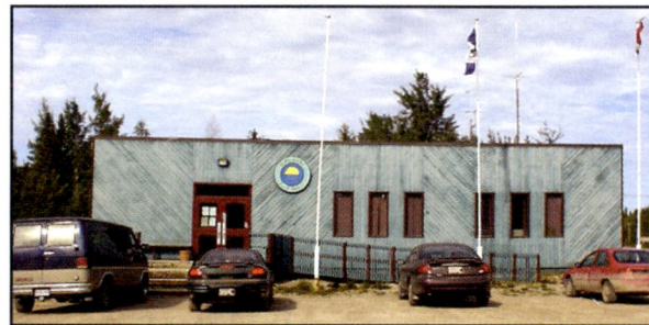
K'at'l'odeeche First Nation Administration Centre
