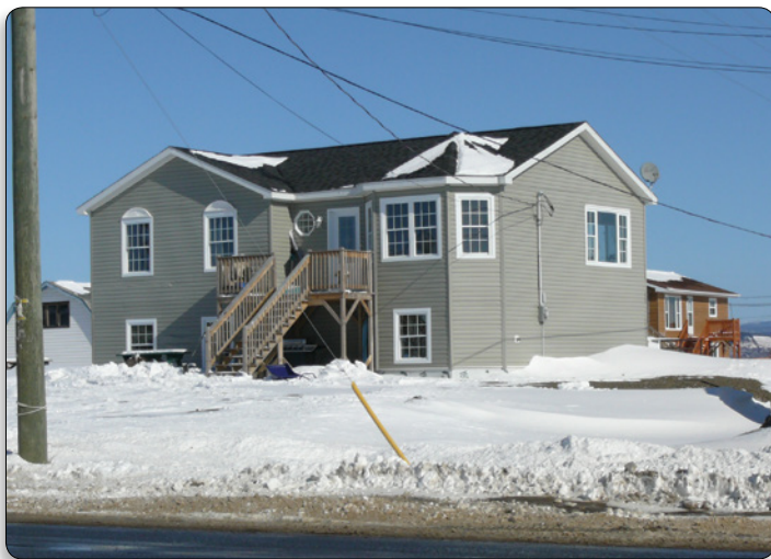
Figure 3 Newly built home with improved site conditions - the house is built on higher ground and was completed after conducting site inspections during construction.
