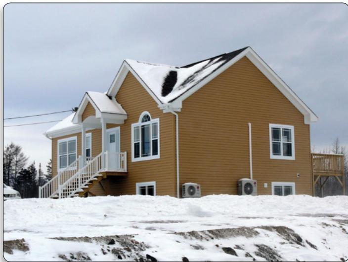
Figure 2 A newly built home with mini-split compressors on the exterior—one for the basement area and the other for the upstairs. Worthy of note is the height of grade built up above the level of the road and the height of the foundation out of the ground to provide natural light to the lower units.
