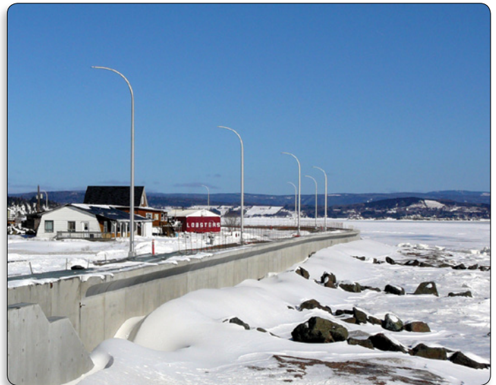
Figure 1 Dike and concrete seawall along the Atlantic Ocean shoreline of the community built after an ocean surge caused by a severe storm flooded houses in 2010.
