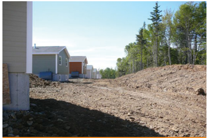
Figure 4 Improved surface drainage behind the hillside houses
