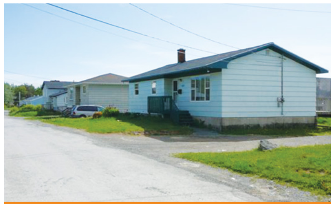
Figure 1 Housing in Membertou First Nation
