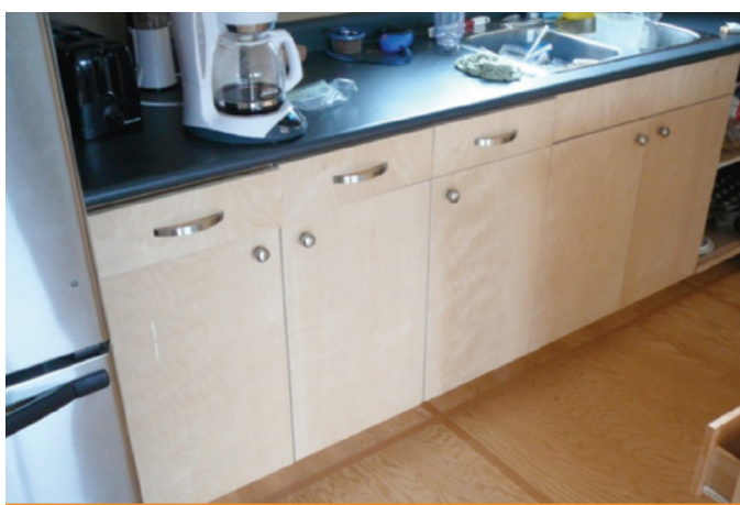
Figure 7 Mold remediated house showcasing locally made kitchen cabinets and varnished plywood floor
