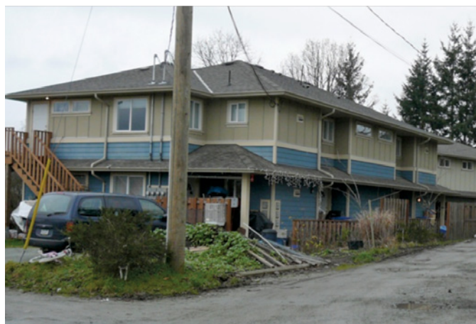
Figure 5 Newly constructed back-to-back fourplexes in Tsartlip
