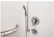
» Height-adjustable, hand-held shower on slide bar with long hose and shut-off valve
