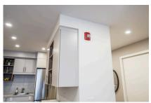
» Visual alarm connected to the building's fire alarm panel
