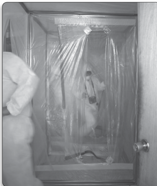
Isolate the work area to protect the occupants
