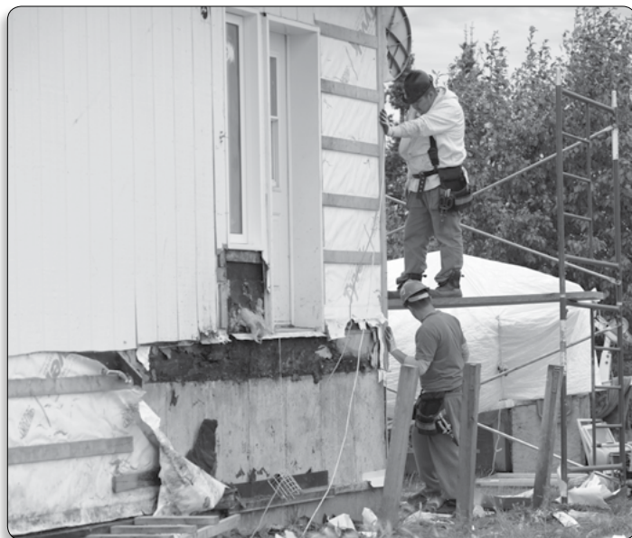
Trained contractors repairing water damage
