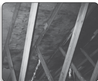
Discoloration and staining on the underside of the roof indicates a water leak
