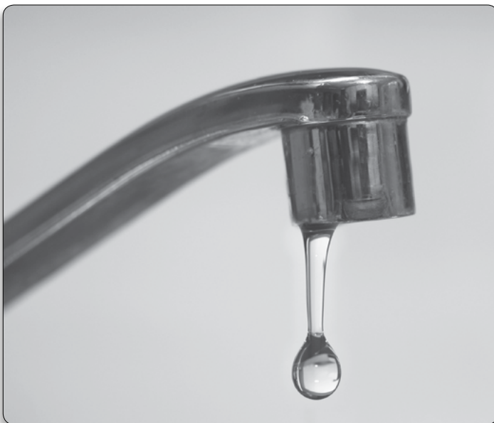
Dripping faucets add to humidity problems
