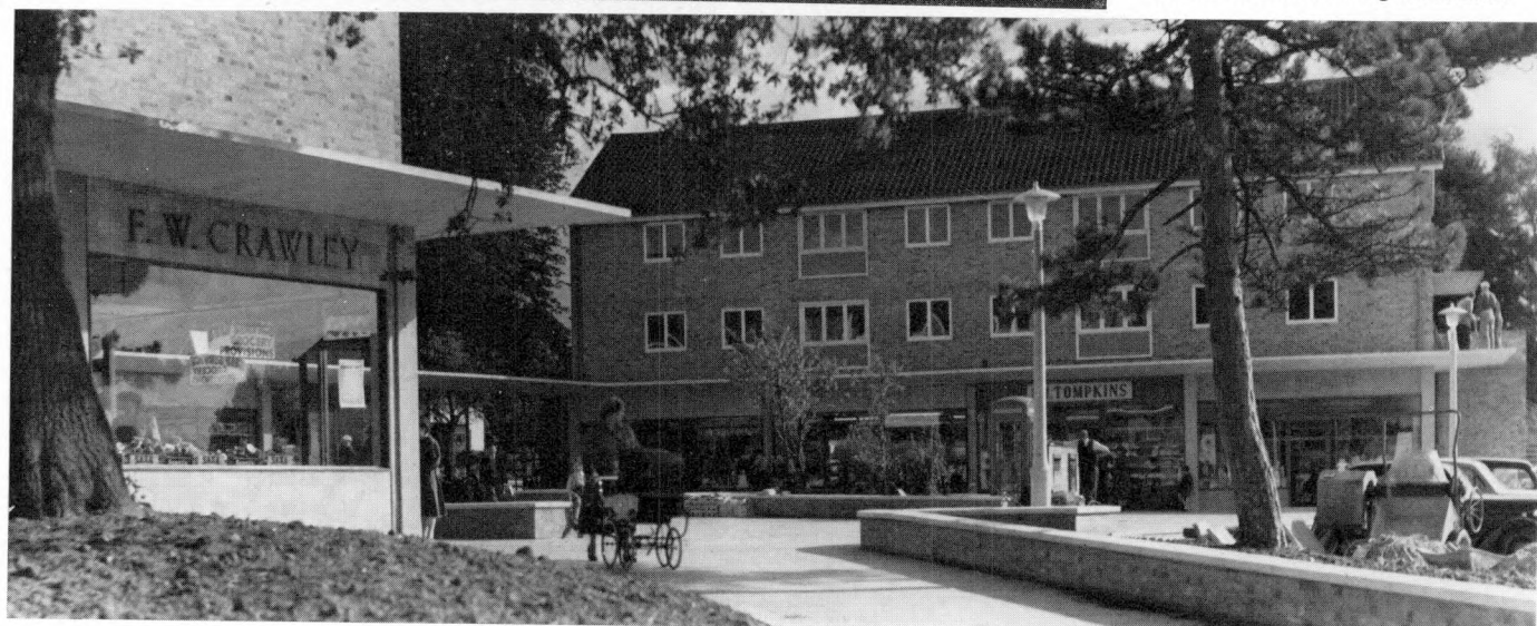
5 The first of the neighbourhood shopping centres built: Priestwood Square with ten shops and flats above just after its completion in 1954
