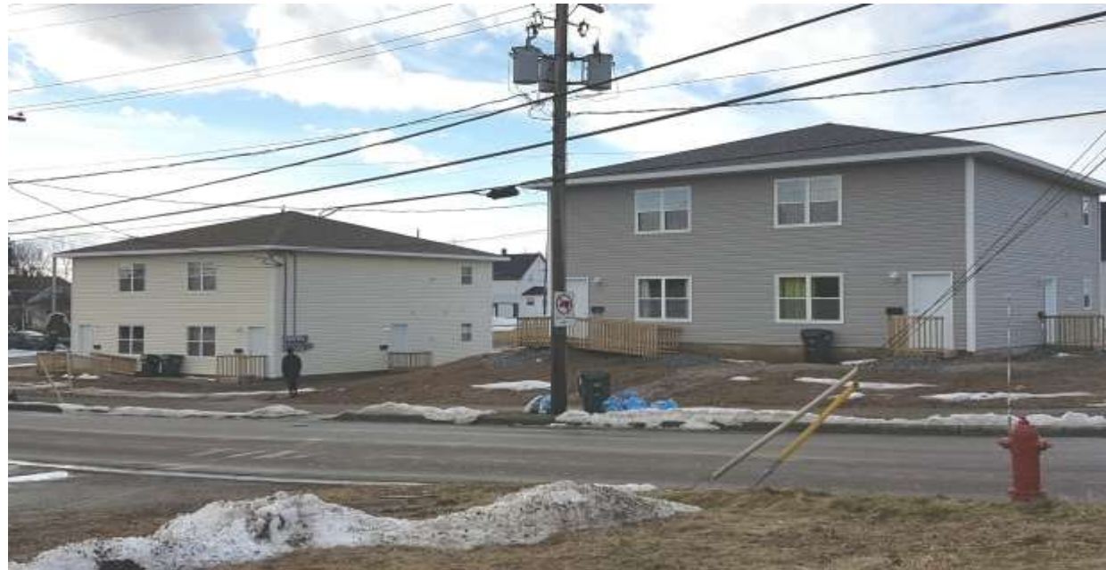
Photo credit: George Mortimer/CBC photo
